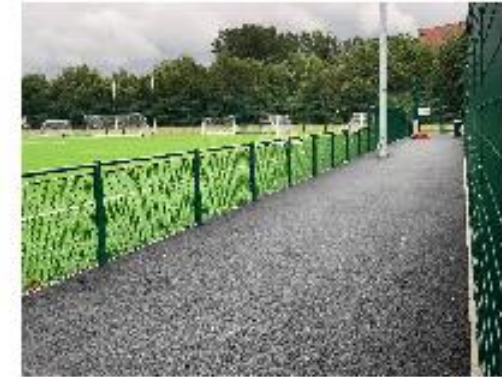
Porous macadam hardstanding to side of pitch
