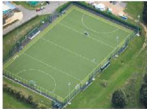
Sand dressed synthetic turf, its appearance similar to well-maintained natural grass
