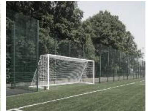
Rigid panel ballstop fencing to perimeter of facilities, powder coated RAL 6005 dark green so discrete against a rural backdrop
