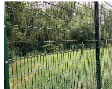
Rigid panel ballstop fencing to perimeter of facilities, powder coated RAL 6005 dark green so discrete against a rural backdrop
